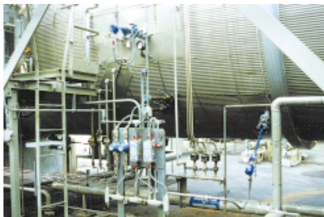
Fig. 1. Energy absorption probes system installed on an electrostatic dehydrator (desalter) for interface control.
